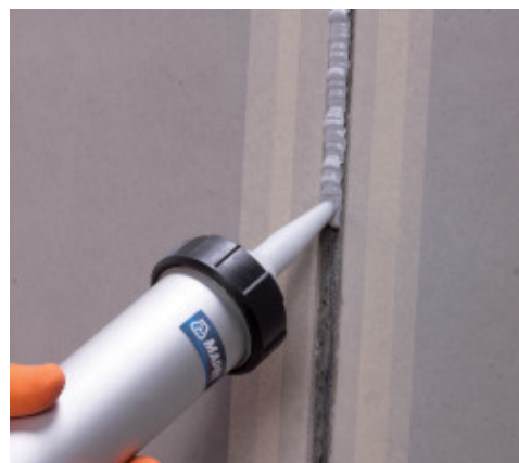
Application de Mapeflex PU40
